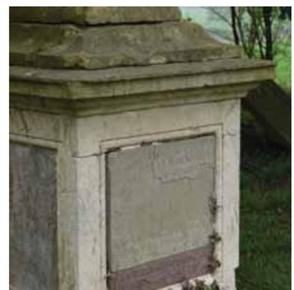
Appropriate methods and materials for repair are essential. In particular, any new metal fixings must be non-ferrous, and an appropriate lime mortar must be used. Vegetation needs to be removed thoroughly but with care, and this may involve at least partially dismantling the tomb in order to get at all root growth out. The use of weedkiller will in most cases not be appropriate, as it poses problems for wildlife, and its effects over a period of time may in fact damage the stonework of the tomb.
